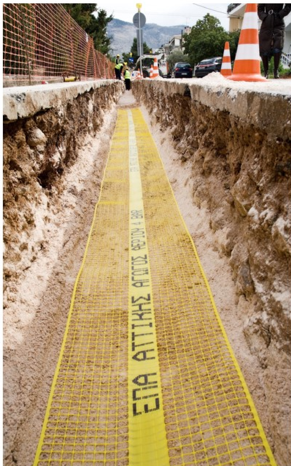
7. Marking grid installed
