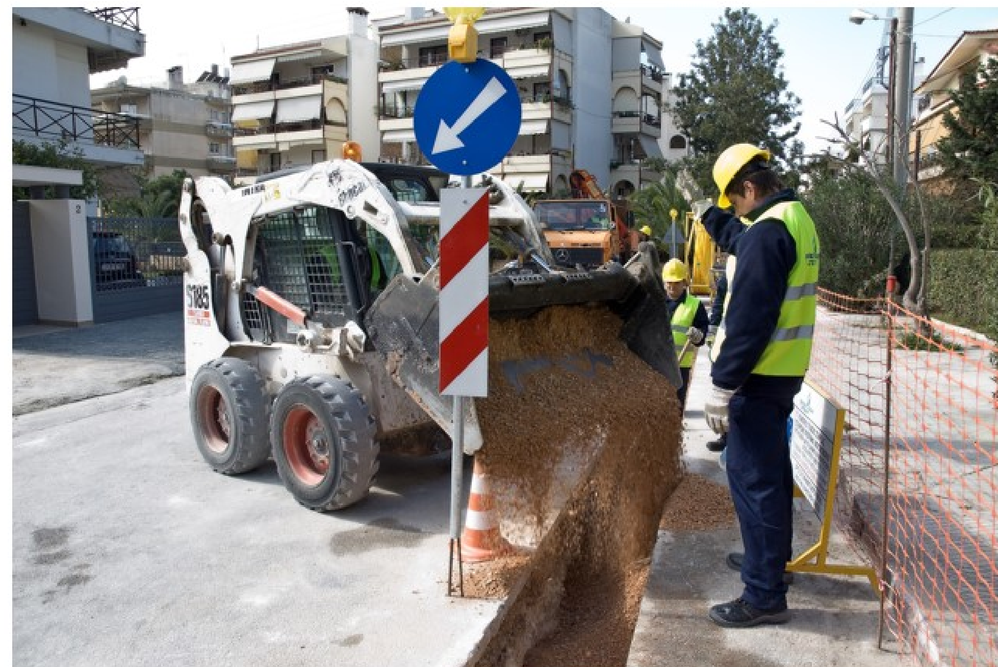
8. Trench backfilling above marking grid with aggregates (3A)
