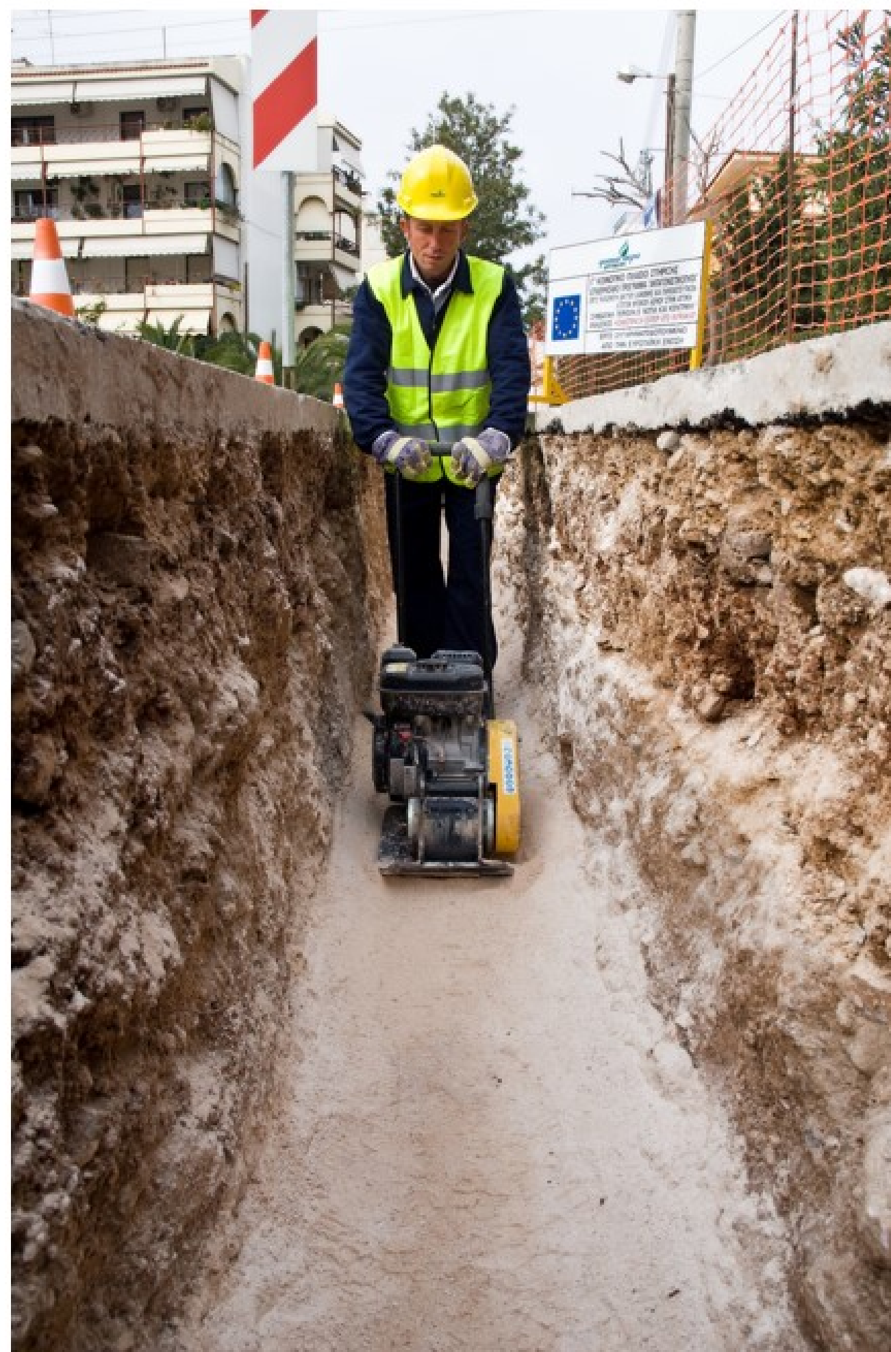
1. Sand Compression below the pipe
