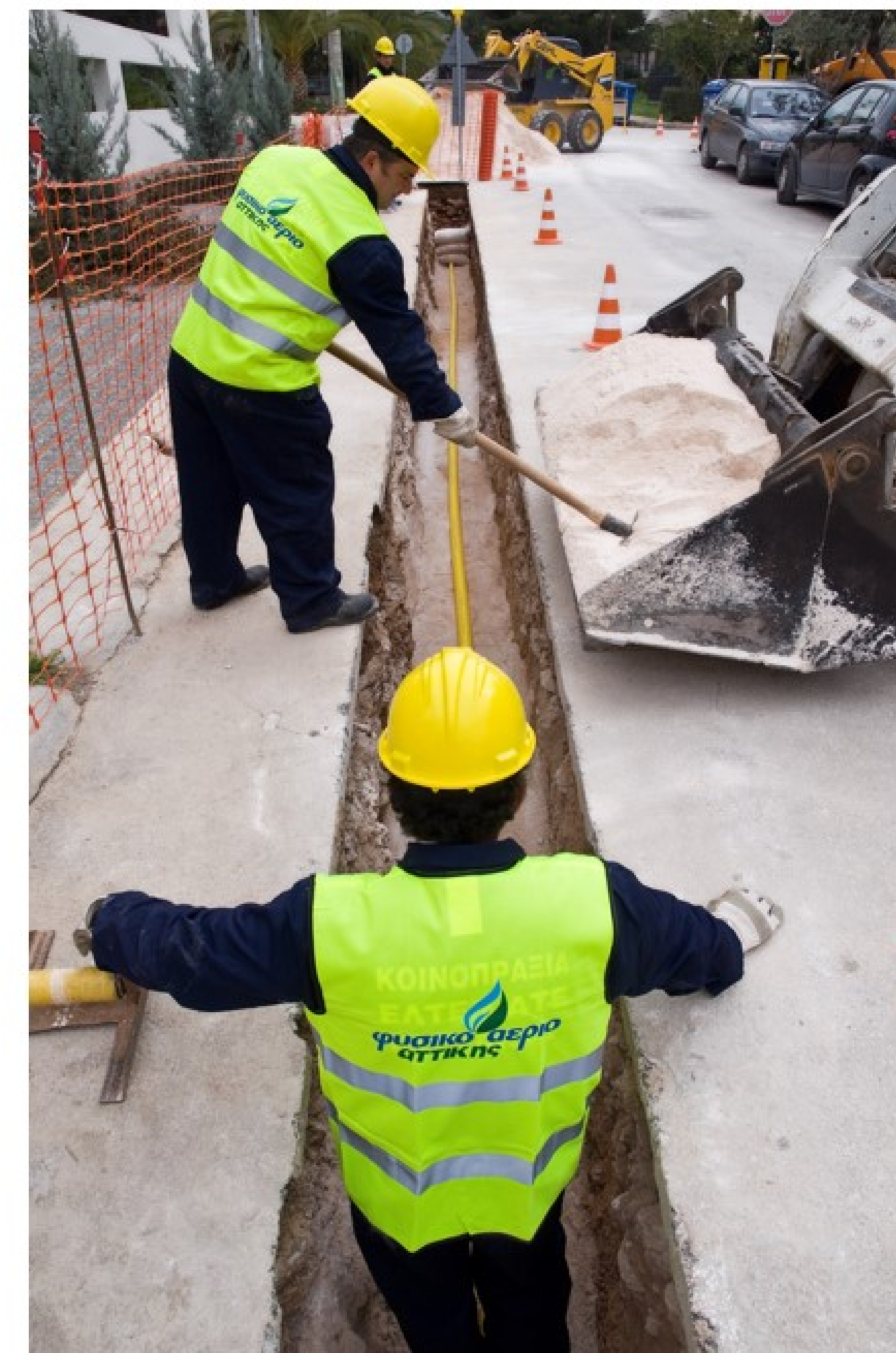
3. Pipe backfilling with sand
