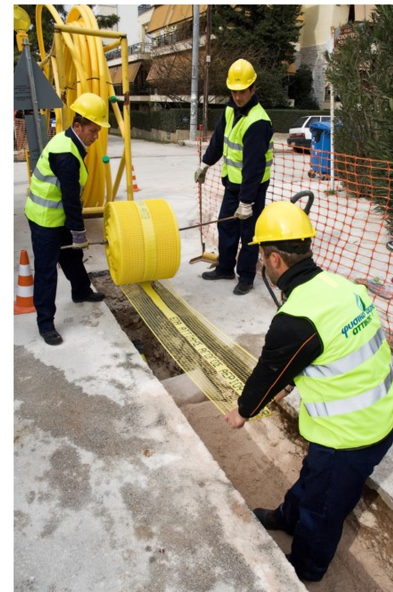
7. Marking grid installation
